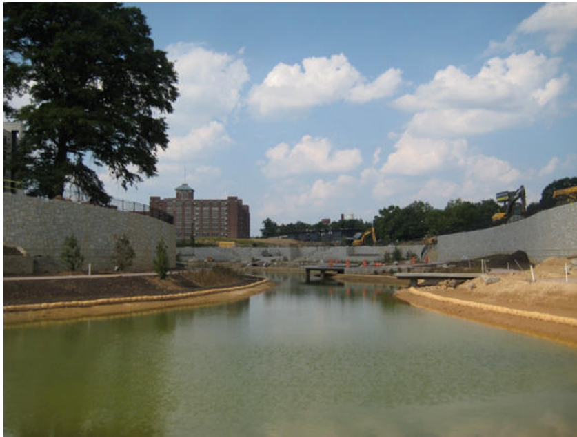
Fig. 4: Detention pond in Old Fourth Ward Park (2010)
