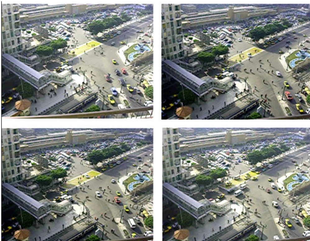
Fig. 9: Different shots showing the new situation after using the pedestrian bridge which reflects the existing situation.
