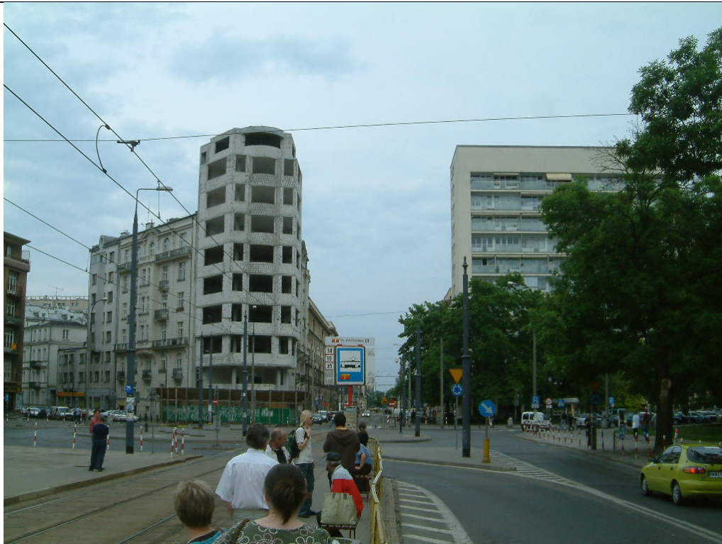
Fig. 4: An example of the “good neighborhood rule”. Warsaw, Politechniki square. The building is still under construction. Photo: Michał Beim
