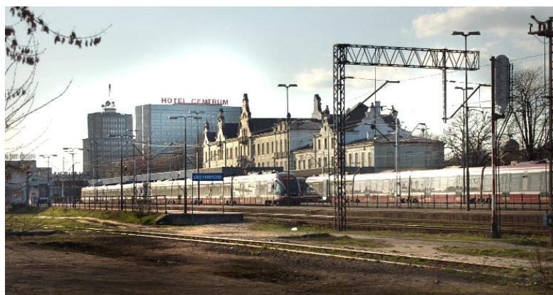
Fig. 10: Old railway station which is going to be redeveloped and hidden underground. Photo: M.Hanzl
