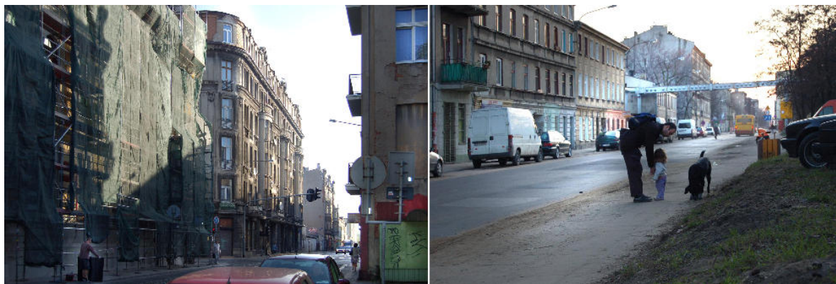
Fig. 6: Direct neighbourhood of the project area: Kilińskiego Street (on the left) and Tuwima Street. Photo: M. Hanzl
