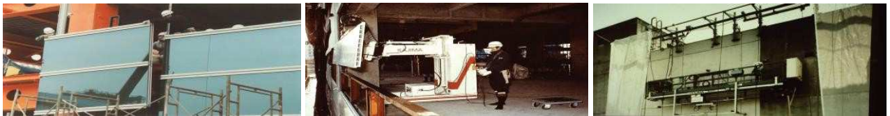
Fig. 19 (left): Panels' installation system mounted to the roof (Kajima, 2016). Fig. 20 (middle): Panels' installation on-floor system (Kajima,2016). Fig. 21 (right): Façade painting system (Kajima, 2016).
