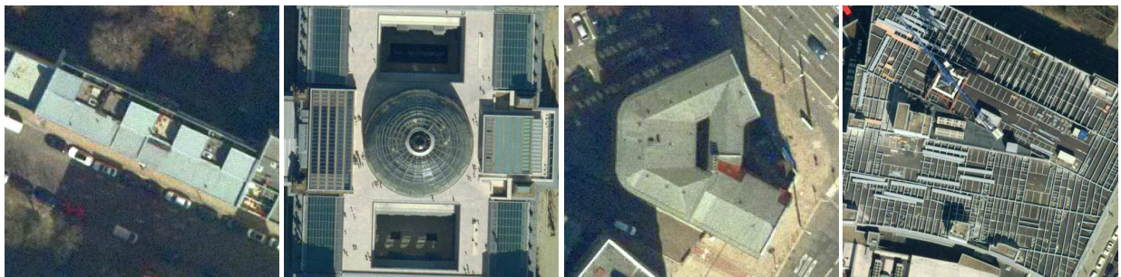
Fig. 13: Roof extensions - 8a) housing, solid wood construction, 8b) Bundestag dome, steel and glass, 8c) Metropolitan School, timber frame construction 8d) Hotel, prefabricated wooden boxes (under construction).
