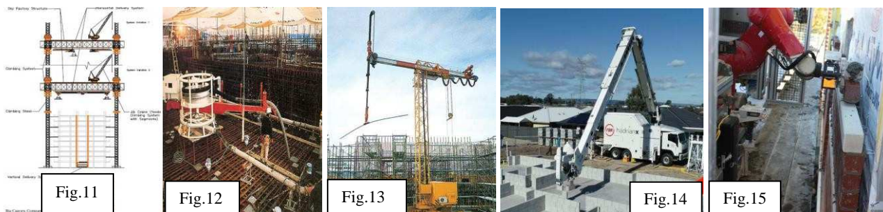
Fig. 11: Obayashi on-site factory (Bock, 2016). Fig. 12: Concrete casting robot (Kajima, 2016). Fig. 13: Reinforcement positioning crane (Takenaka, 2016). Fig. 14: Hadrian system (fastbrick, 2021). Fig. 15: SAM100 (construction robotics, 2021).
